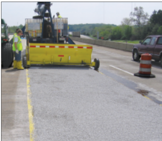
Left: Installation of the overlay
