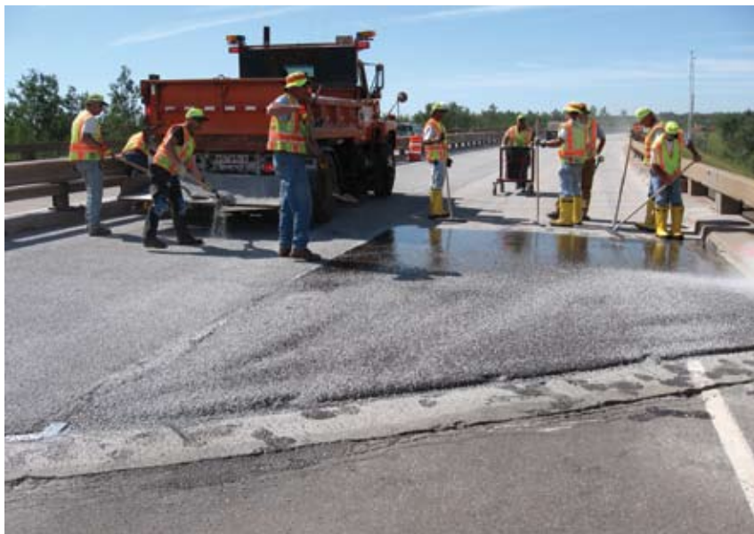
Fig. 2: Aggregate is broadcast over the initial epoxy layer
